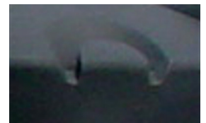
Lower fitting is a 2" bulkhead.
