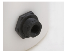
Lower fitting is a 2" bulkhead.
