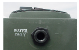
Top fitting is a 1-1/2" polypropylene bulkhead fitting for float valves.
